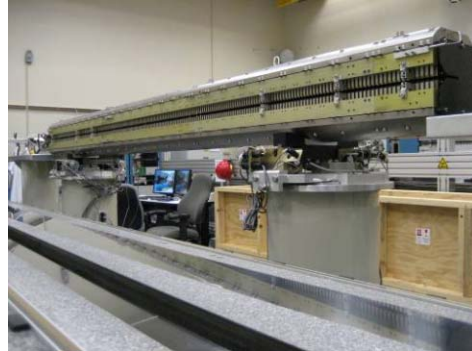
Figure 1: Rough tuning bench showing an LCLS undulator on the cam mover system.
